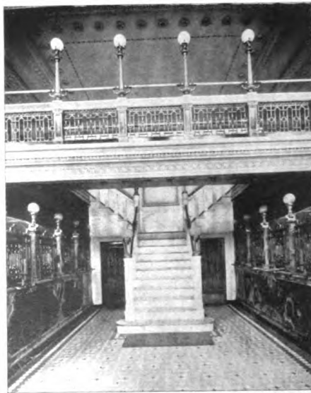
Staircase Leading to the Mezzanine Floor.
